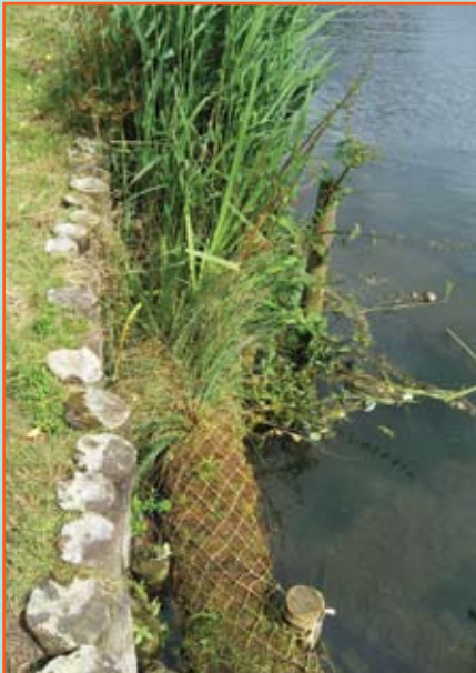
Planted coir rolls can provide vegetation along banks.
